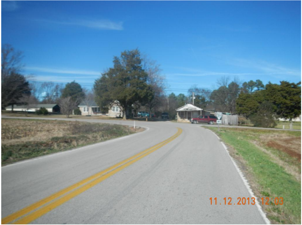
Photograph 1 – DSCN2080. N35.0521°, W-86.2578°. View facing north of SR-97 near STA 12+00. Beans Creek Rd joins from the right.
